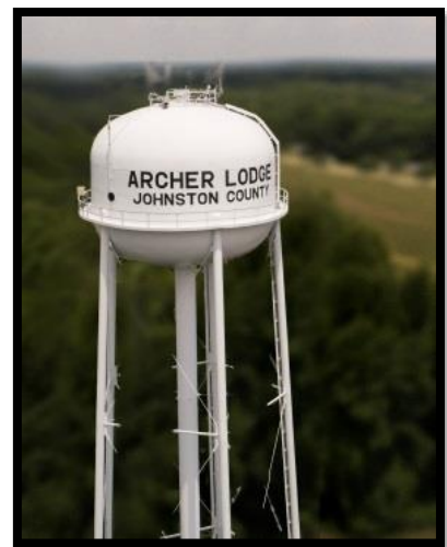
Archer Lodge Water Tower (Archer Lodge, 2019)
